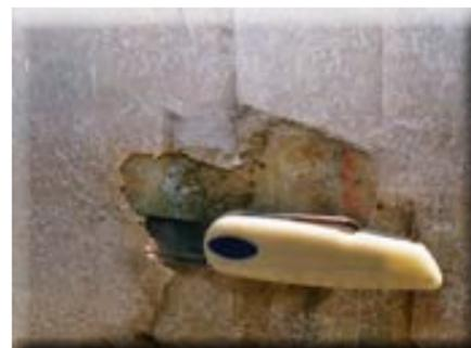
Massive damage incl. delamination, Area must be rebuilt with fiberglass fabric or scrim
