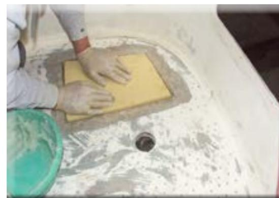
Sandwich structures are repaired. Here: The replacement of a complete sandwich structure and resin injection in combination
