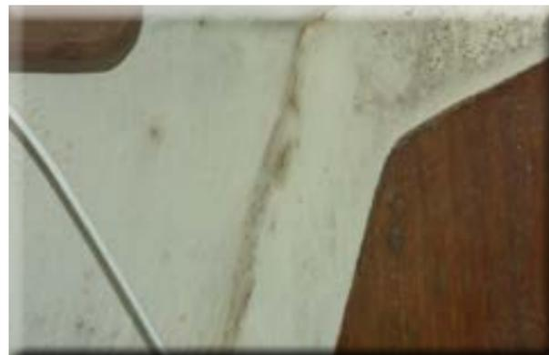
Cracks in the corners
