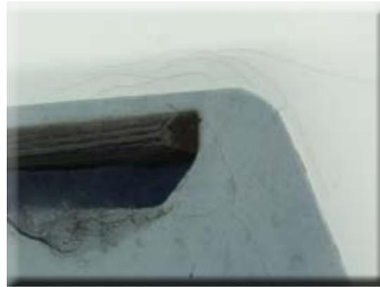
Cracks and holes in the gelcoat
